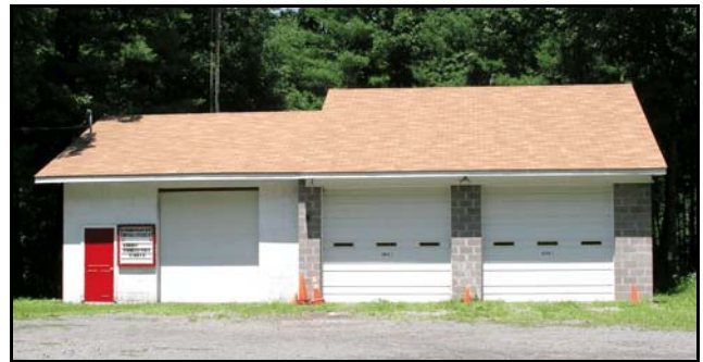
Blooming Grove Substation
