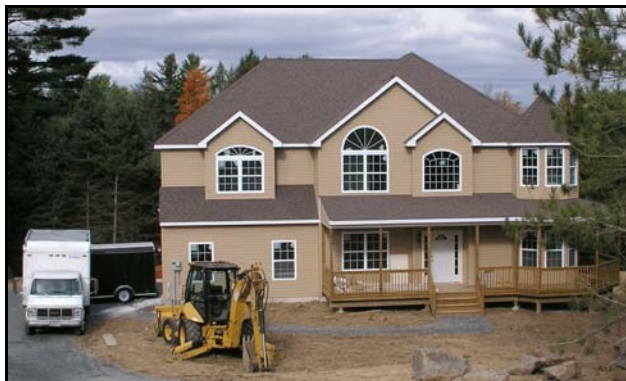
Recent Home Construction
