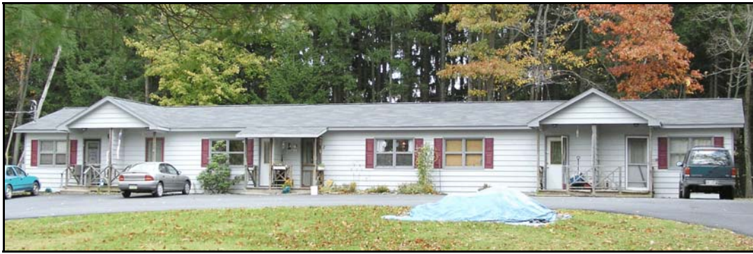
Apartments Along Route 390
