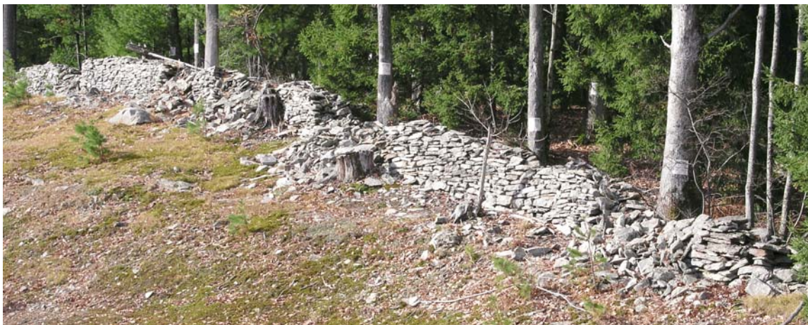
Stone Wall Along Route 739 in Commercial Zoning District
