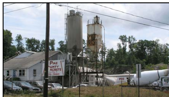
Pike County Concrete
