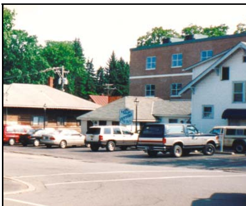
Before Streetscape Improvements
