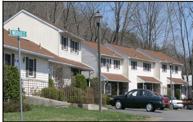
Townhouses, Wheatfield Village, Milford Township
