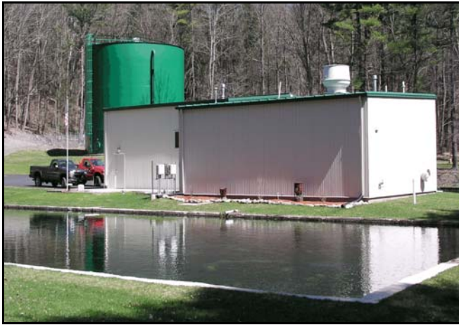
Milford Water Treatment Plant and Storage Tank
