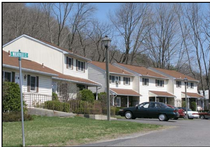
Townhouses, Wheatfield Village, Milford Township
