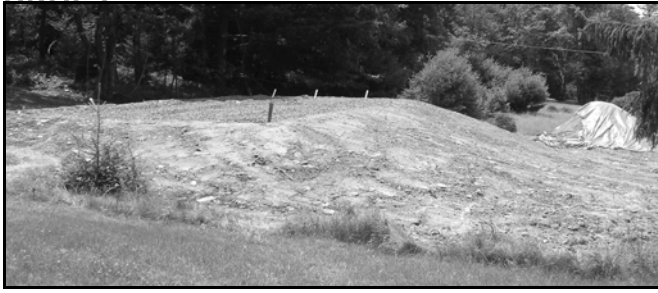
Sand Mound Under Construction
