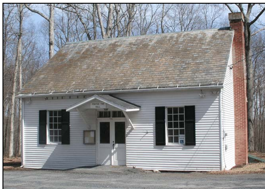
Porter Township Building
