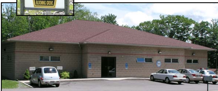
State Police Barracks, Route 402
