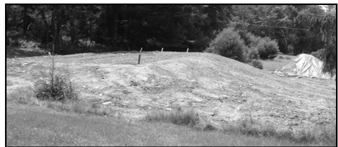
Sand Mound Under Construction
