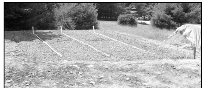
Sand Mound Under Construction
