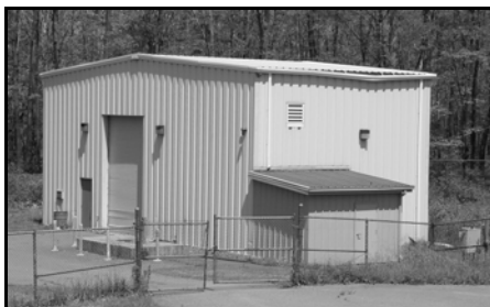
PennDOT I-84 Sewage Treatment Plant
