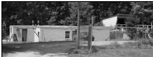
Wallenpaupack Area School District Sewage Treatment Plant
